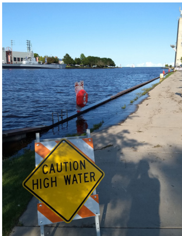
Vulnerability assessments to identify critical infrastructure can help communities adapt to periods of high and low water levels along the Great Lakes. High water levels overtop a seawall and inundate a sidewalk in Manitowoc, Wis. Photo credit: Adam Bechle, Wisconsin Sea Grant
