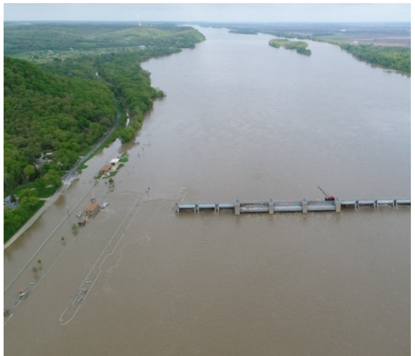
Flooding has caused damage to transportation infrastructure on the Mississippi River. Mississippi River lock and dam under water during 2019 flood in the Rock Island District, Iowa. Photo Credit: United States Army Corps of Engineers
