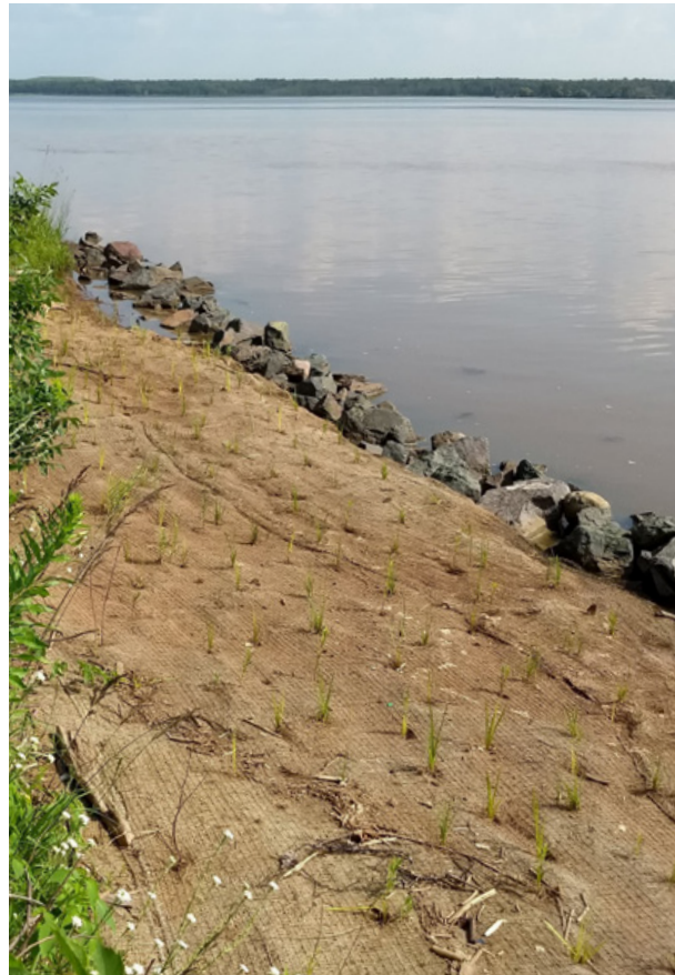
Nature-based solutions can protect shorelines and, once established, be more appealing and beneficial for wildlife. Rock sill and marsh vegetation plugs installed to protect the Wisconsin Point shoreline in Allouez Bay, Superior, Wis. Photo credit: Adam Bechle
